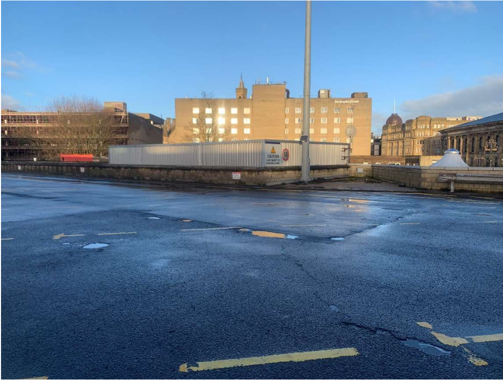
Photo 90- Cracks in tarmac surface
