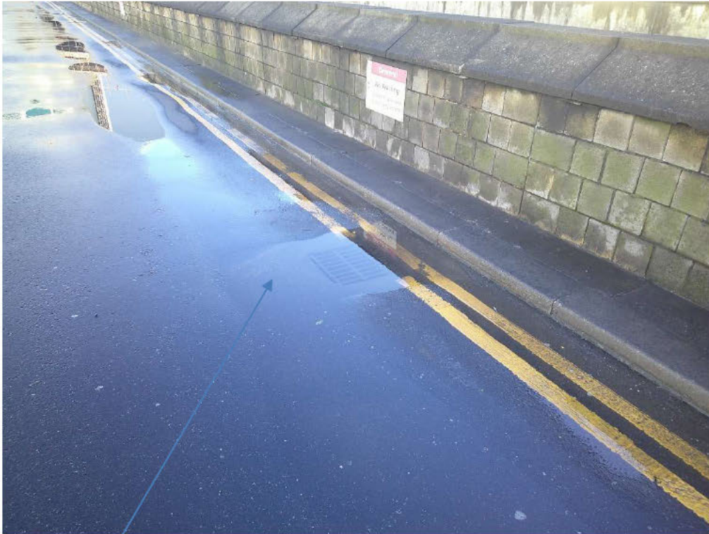
Photo 96 – Blocked gully
